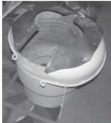
The splash guard unit used in grouting the cable-tool drilled well.
