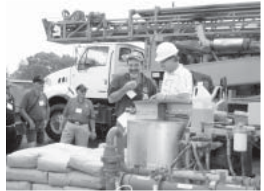
Dennis Duty of Baroid and John Buehler demonstrate how to grout heat pump loops in wells with thermal grout
