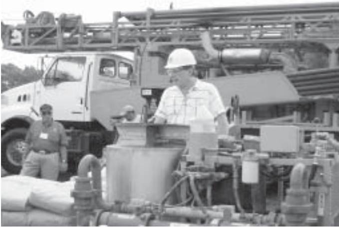
Dennis Duty of Baroid and John Buehler demonstrate how to grout heat pump loops in wells with thermal grout
